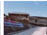
Welfare Education Development Center completed (2003)
